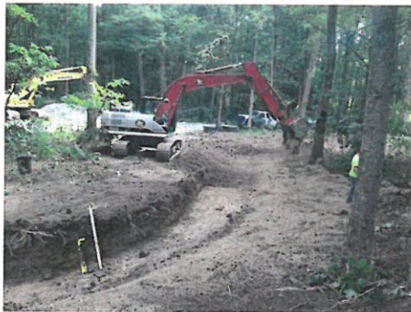
Construction of new stream channel in Tennessee (KCI Technologies)
