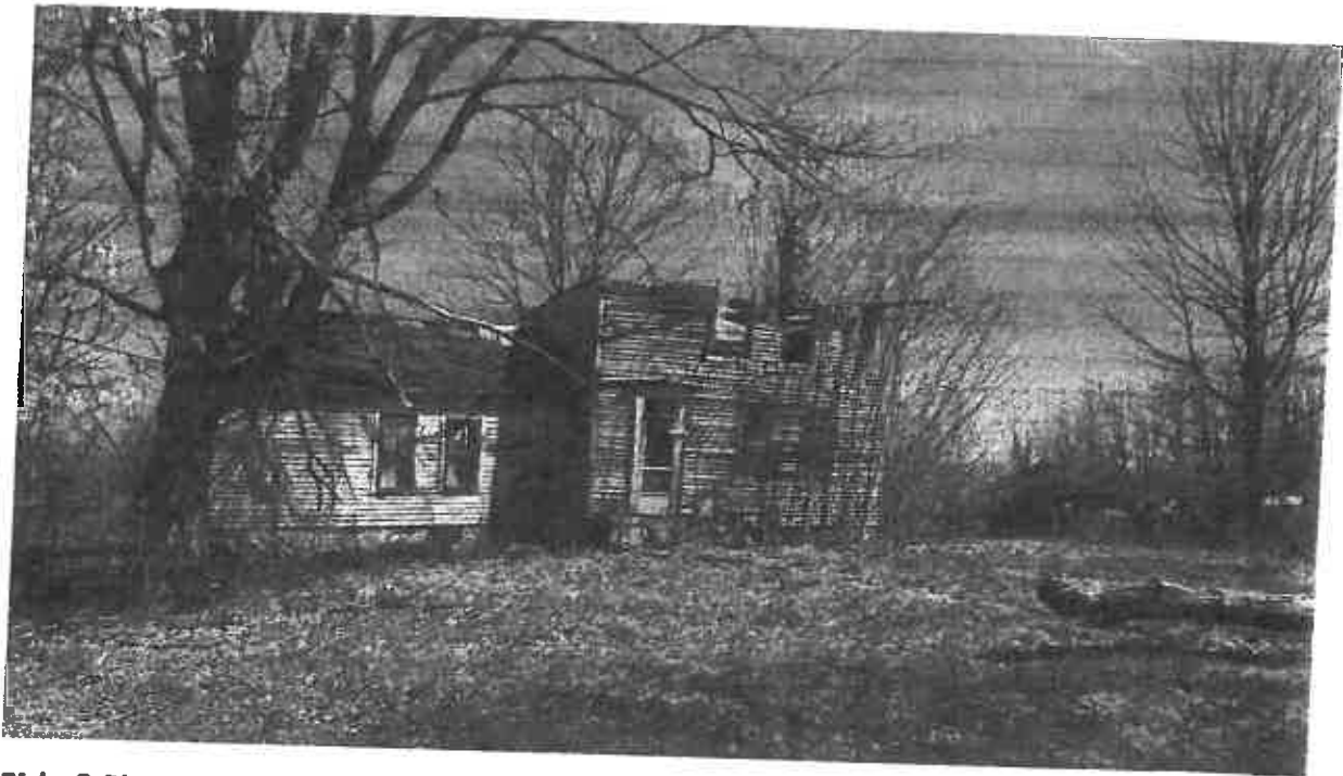
Ricky & Rhonda Deutscher Trustees, 9565 W 100 N, Michigan City, Parcel ID 460528400001000046 (abandoned since at least 2010, roof collapsed in 2021)
